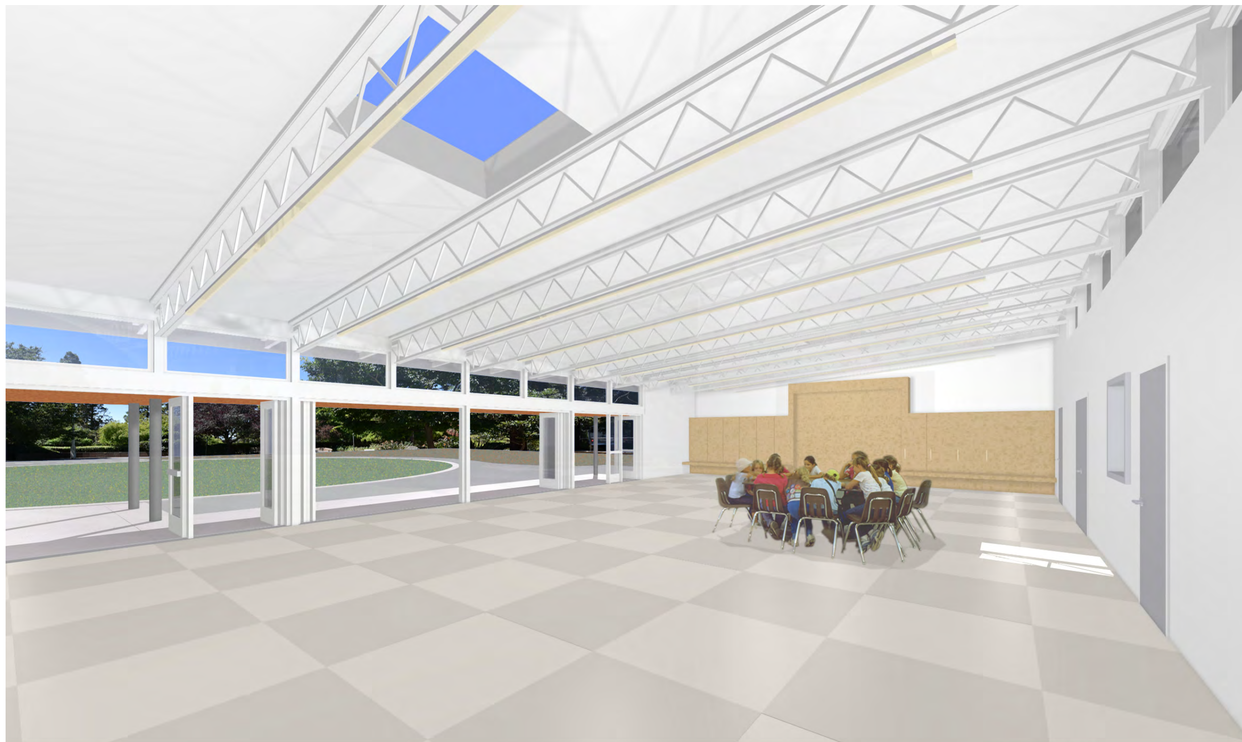
Interior - New Structural Frame, Canopy and Window Wall with NanaWall-Type Doors
