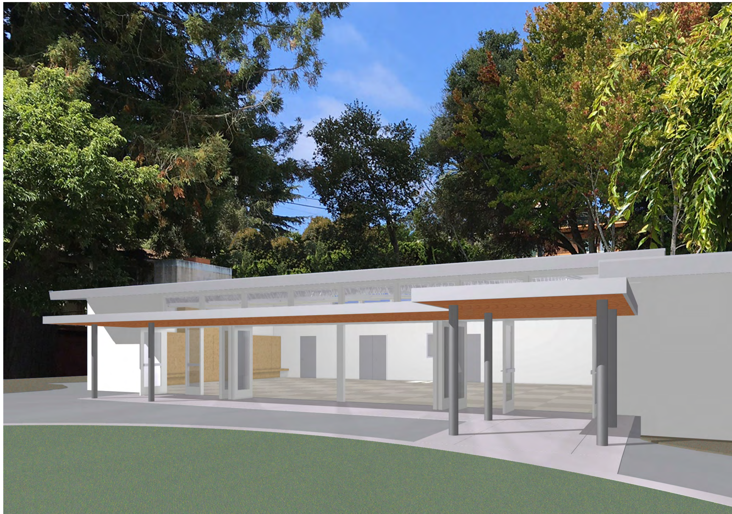
Exterior - New Structural Frame, Canopy and Window Wall with NanaWall-Type Doors
