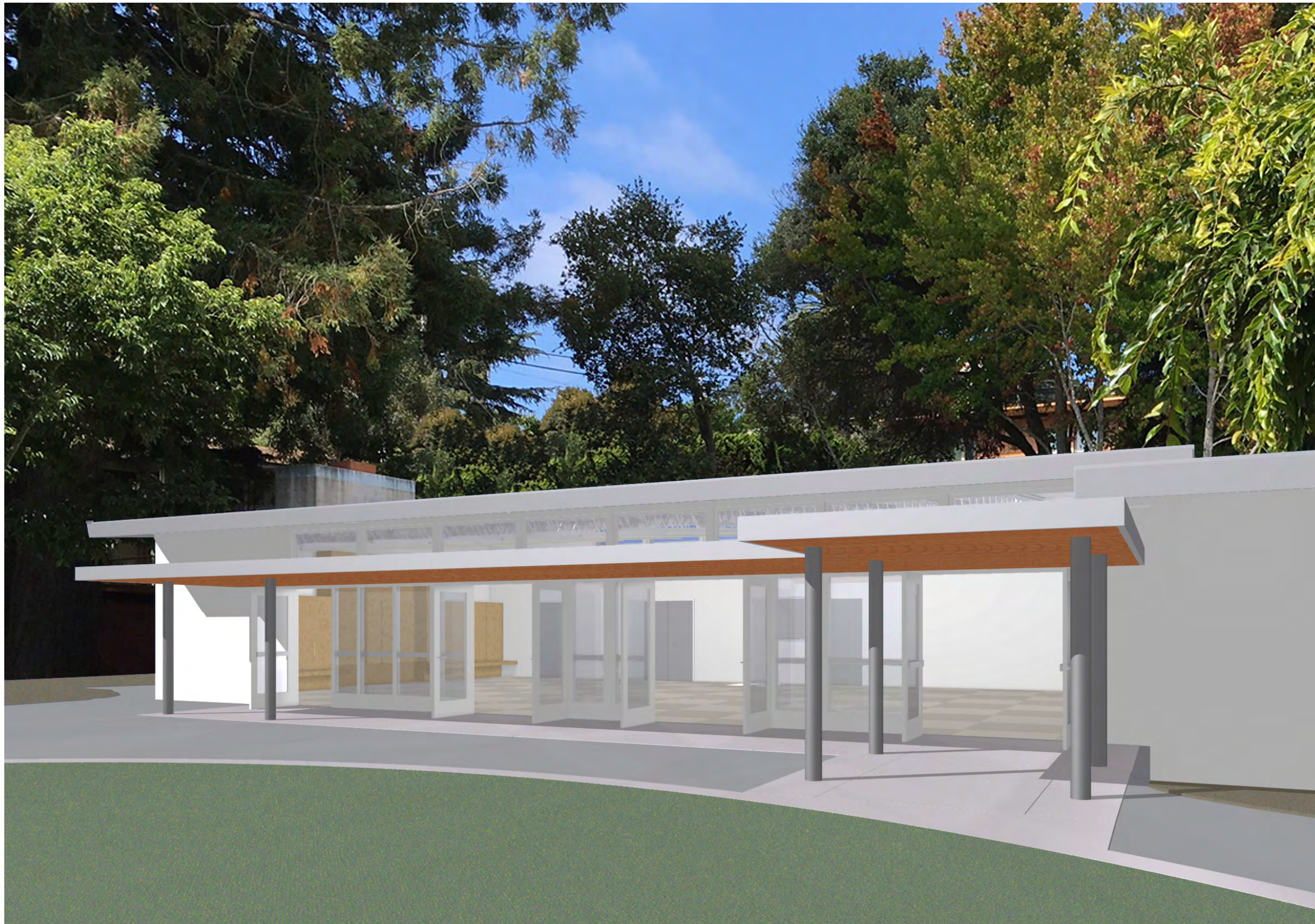
Exterior - New Structural Frame, Canopy and Window Wall with French Doors
